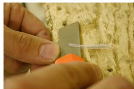
2.3-Trim the nylon tubing 2 inches from one end using an angle cut. This will make it easier to feed the nylon tube through the holes;
